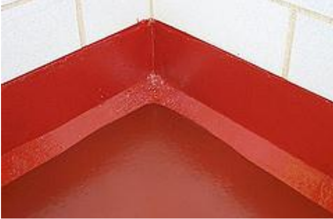
Canted cove-to-wall base, skillfully installed using FloroCrete.
